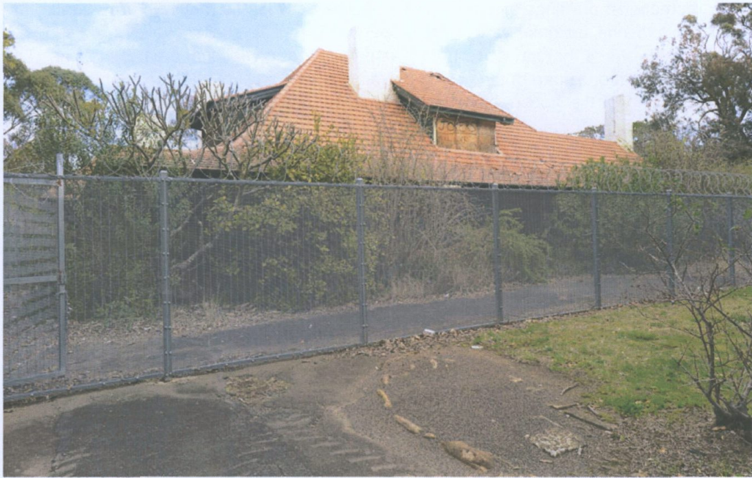
Figure 32 View of house from frontage. While the fence is necessary to provide some security, the generally degraded character of the frontage can be seen with failed pavements. It is noted that the planting around the house has been largely removed in recent maintenance works. Paul Davies 2014.
