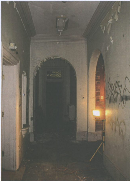
Figure 19 Main hallway looking west. Paul Davies 2014.
