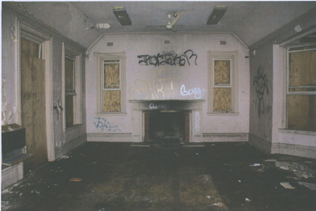
Figure 15 View of room 1 displaying significant vandal damage including evidence of fires and graffiti. The ceiling has been clad in plasterboard. Paul Davies 2014.
