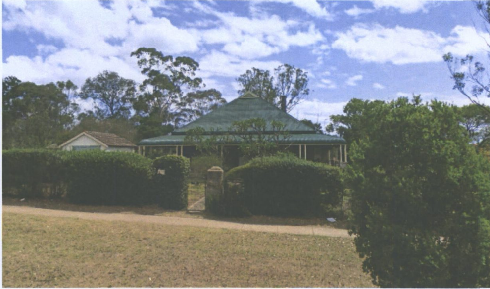
Figure 38 Recent photo of "Woodcrest" at Ingleburn. Rappoport 2010.
