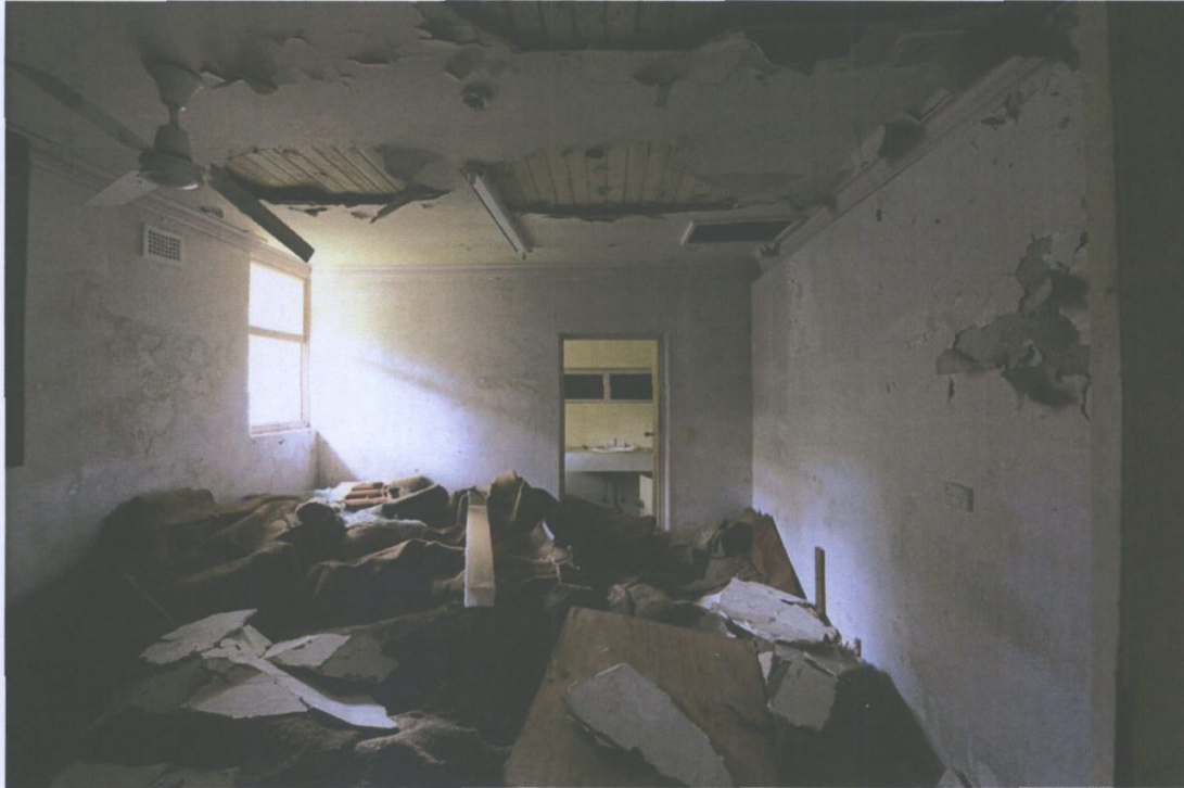
Figure 13 Interior of former garage area, now divided into bathroom and general room. Note the timber boarding above the plaster ceiling and the later joinery from one of the adaptations of this wing for institutional use. Paul Davies 2014.
