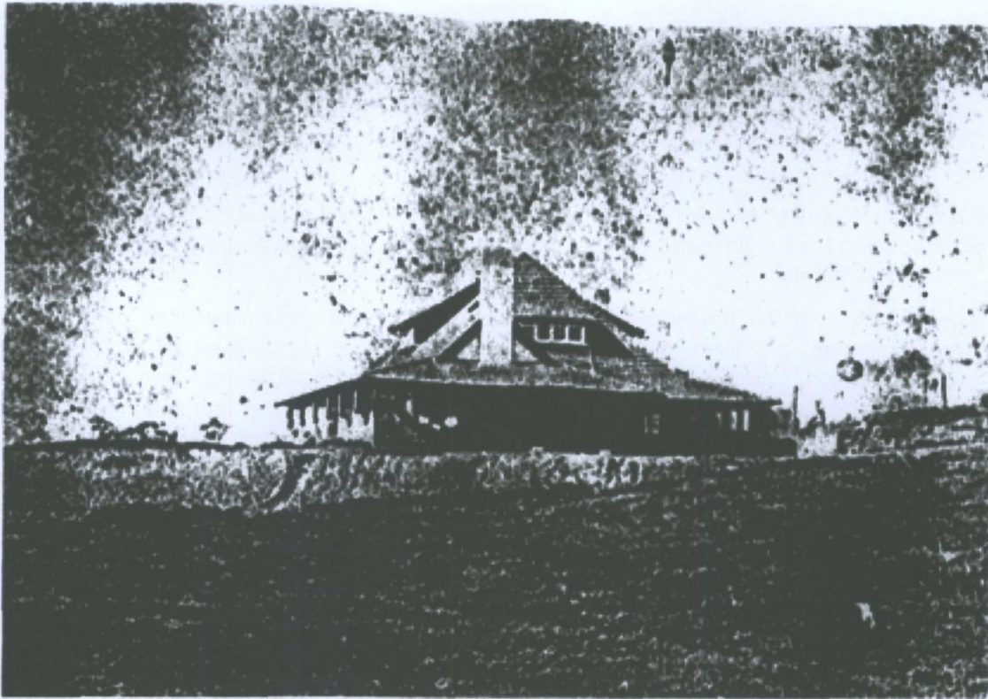
Figure 3 Undated photograph of "Raith" viewed from the north west. The photograph was very likely to have been taken shortly after its completion in 1903. Its original roof configuration and details of dormer fenestration are clearly visible. The site works necessary to provide a level foundation are also quite apparent. (Campbelltown City Library Local Studies Collection).
