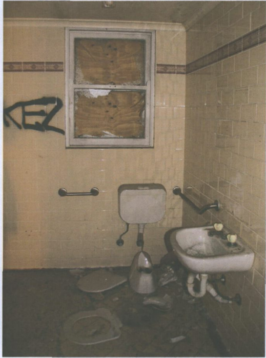
Figure 24 Bathroom 1 facing south. Paul Davies 2014.
